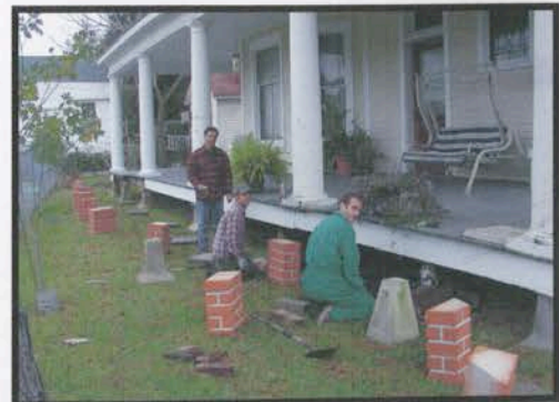
Mark Provost (standing) and employees work on foundation.
