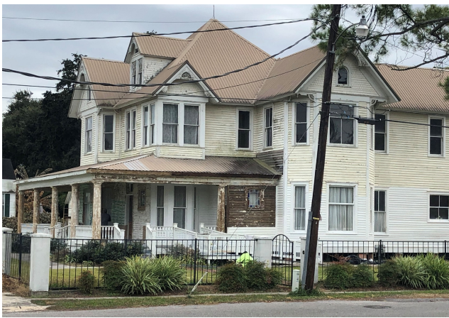
Painting in Progress west side of the House
