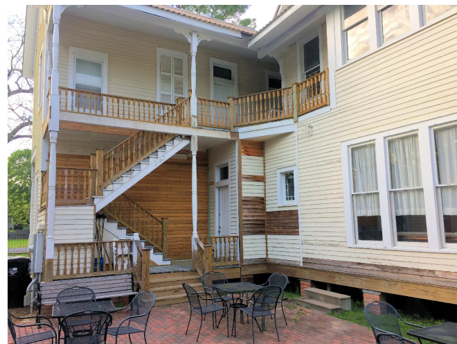
Rear stairs after repair
