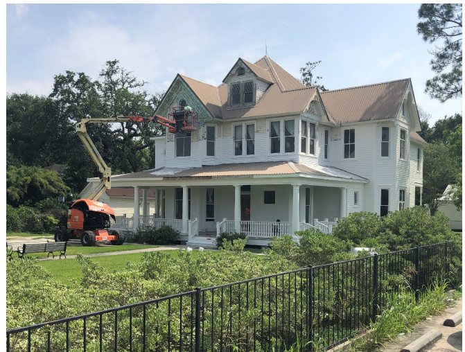
Painting in Progress front view of House
