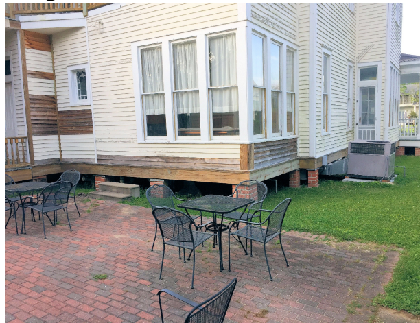
Repairs to the rear of the House
