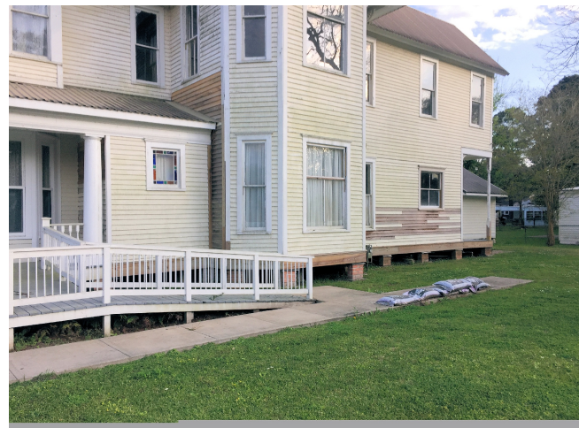
Repairs to the West side of the House
