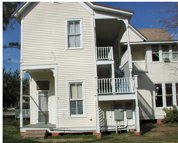
2007 Rear Stairs after repair
